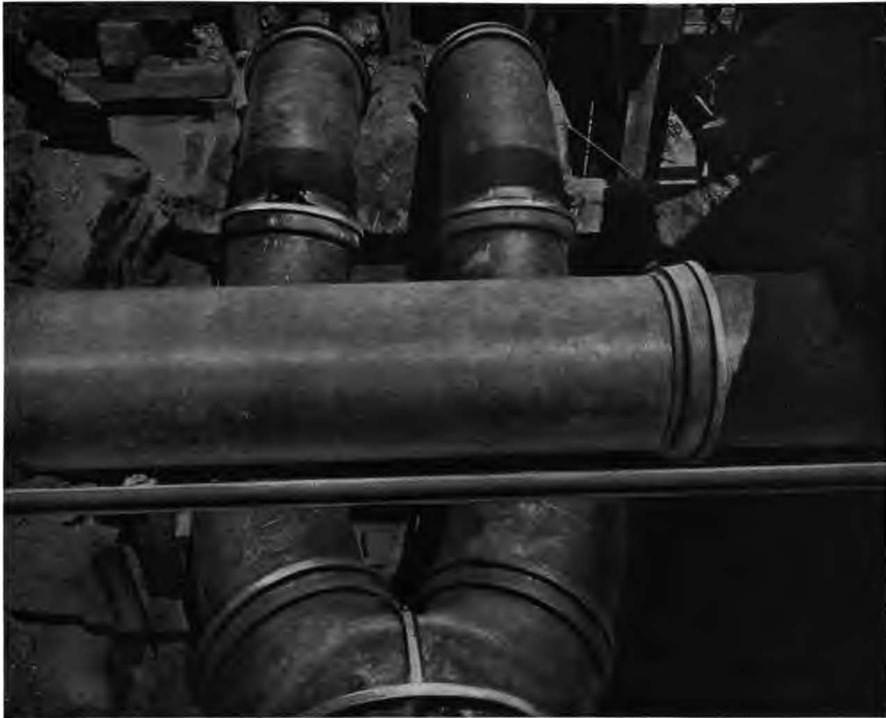
DIFFICULT PIPE WORK—BROADWAY AND 70TH STREET
